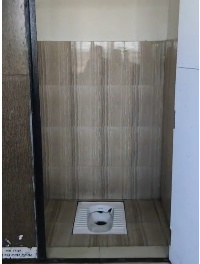
GIRLS TOILET FIRST FLOOR
