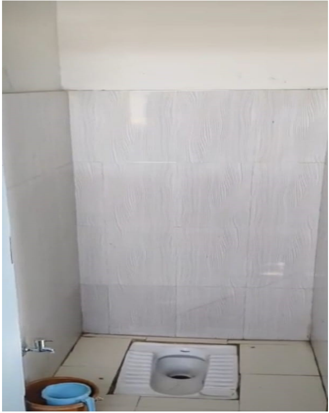
BOYS TOILET GROUND FLOOR
