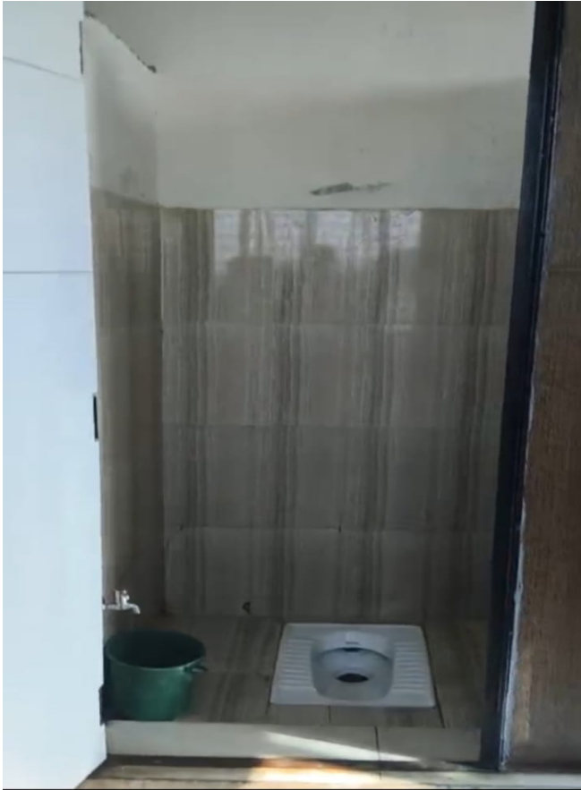
GIRLS TOILET FIRST FLOOR
