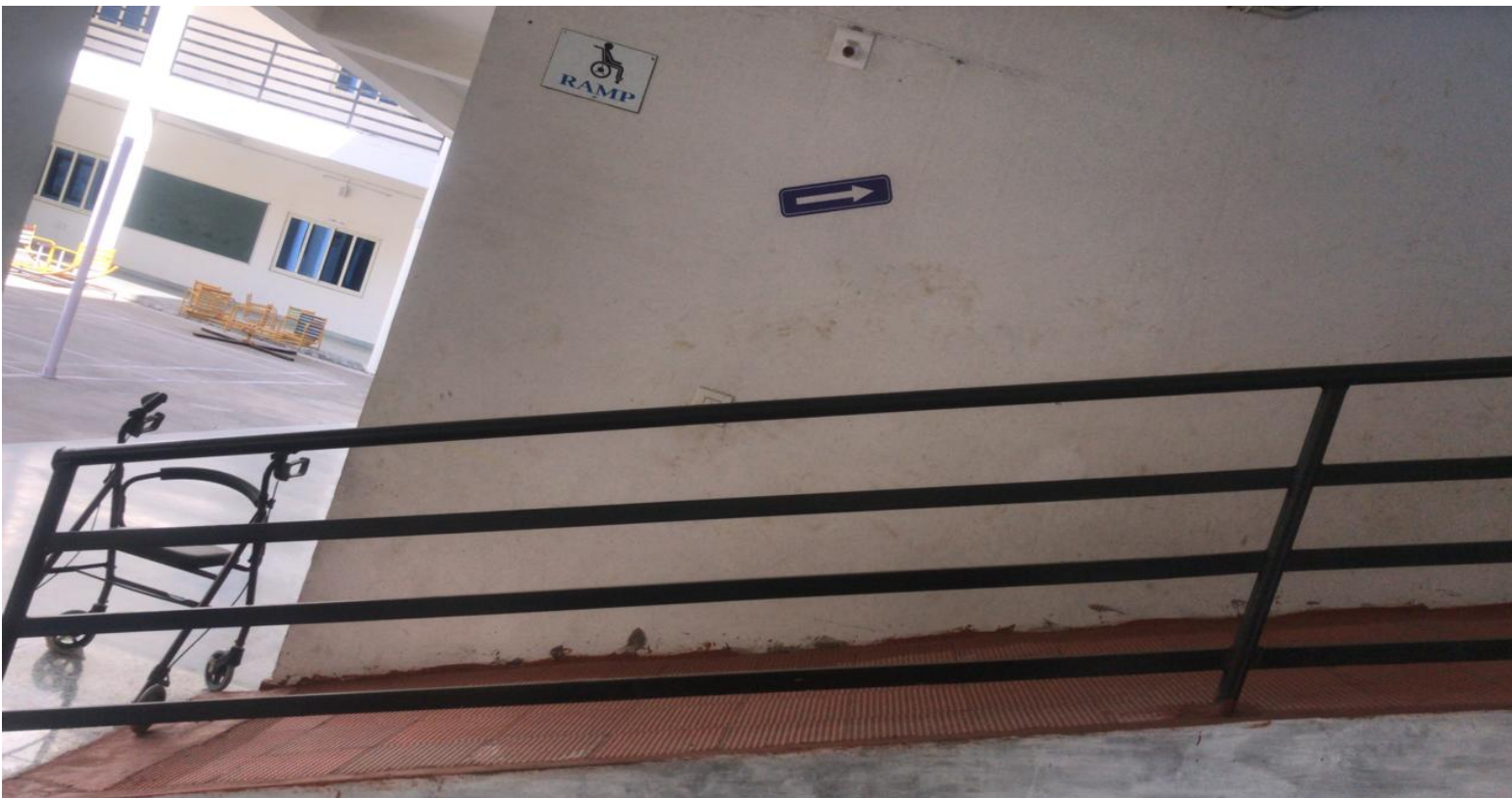
GROUND TO FIRST FLOOR RAMP
